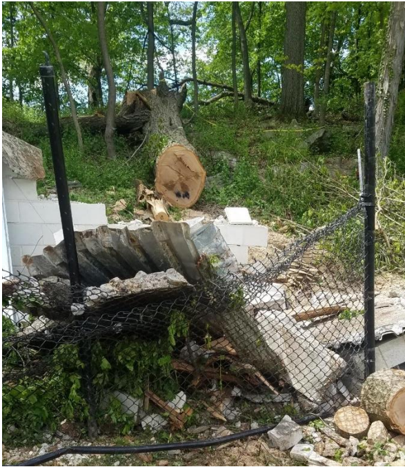
Photo taken by the Village of the tree that failed onto the dugout at Uniontown Park. Although the tree was healthy, its base had significant decay.
